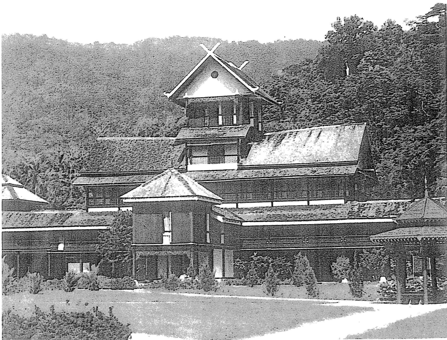
Istana Lama di Seri Menanti, siap dibina pada awal 1900; diperbuat daripada papan tanpa menggunakan walaupun sebatang paku The Old Palace at Seri Menanti, the wooden structure of which was completed early in 1900 without the use of a single metal nail
